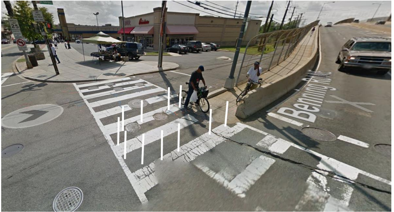
Figure 13: Mock-up of Potential Interim "Pedestrian Refuge" on West Side Crossing of Benning Road.
