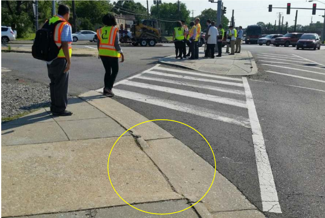
Figure 6. Southeast corner of Suitland Parkway at Firth Sterling Ave SE
