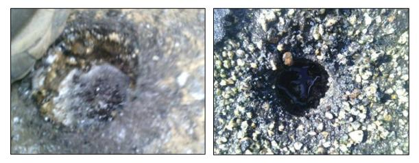
While performing preventative maintenance BLUEFIN identified 238 defects and permanently repaired 91 defects and temporarily repaired 15 defects. BLUEFIN is recommending sections F, V, G, II, FF & EE for immediate replacement. These sections are located in the administration wing of DOC CDF and represent roughly 22,000 sqft of roof area. The areas that we are recommending for immediate replacement are shown below.
