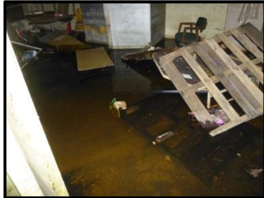
Figure 14 - Flooding (Ground Level)
