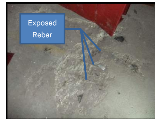
Figure 9 – Exposed Reinforcement
