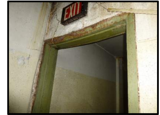
Figure 23 - Rusted Finishing
