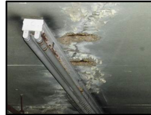
Figure 7 – Exposed Reinforcement
