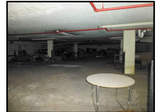
Figure 2 – Ground Level Stored Items
