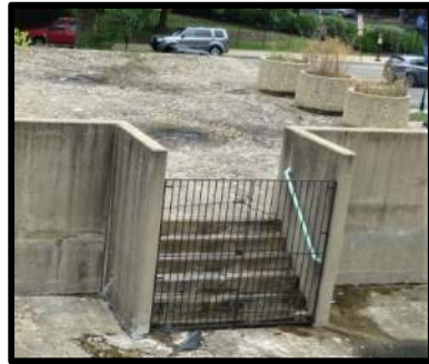
Figure 31 - Upper Roof Topping Slab
