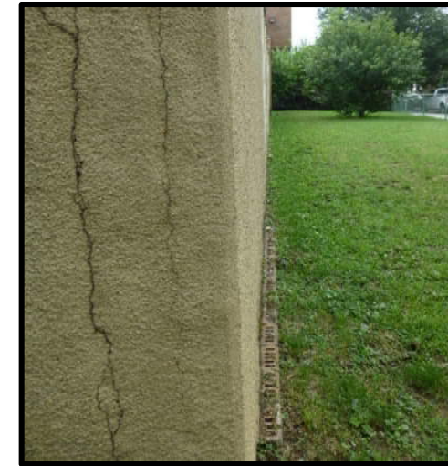
Figure 4 – Parge Coat and Brick Sister Wall
