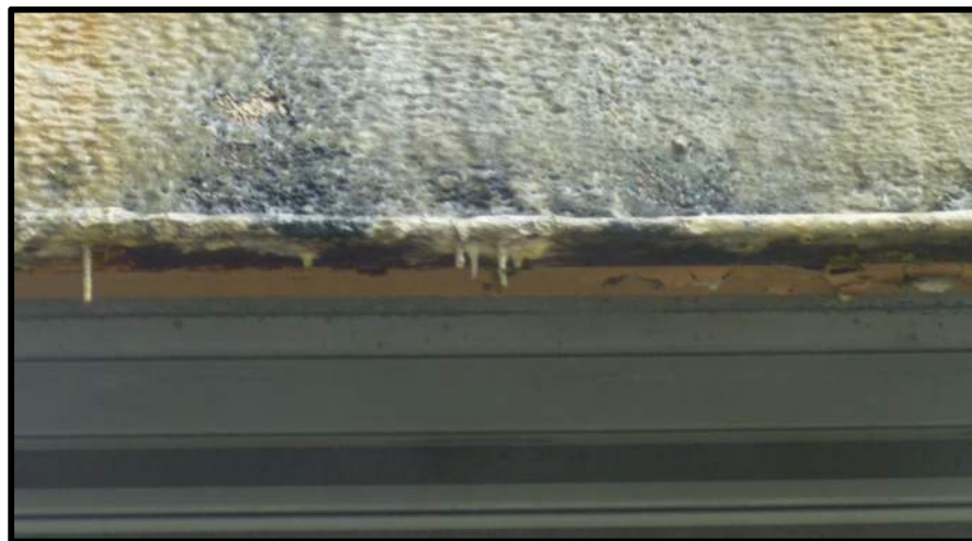
Figure 27 - Rusted Lintel
