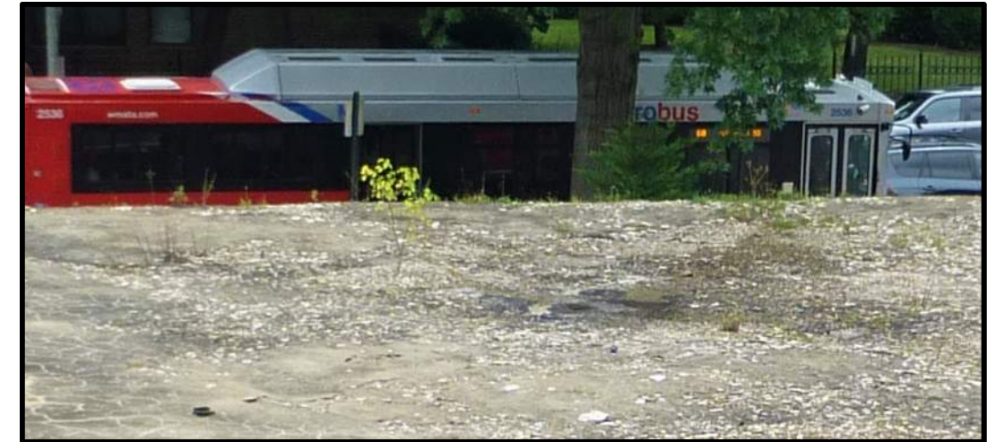
Figure 34 - Vegetation Growth (Upper Roof)
