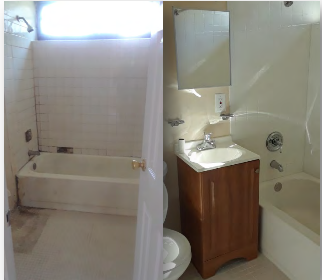
Figure 2. Bathroom at Lincoln Heights, Before and After
