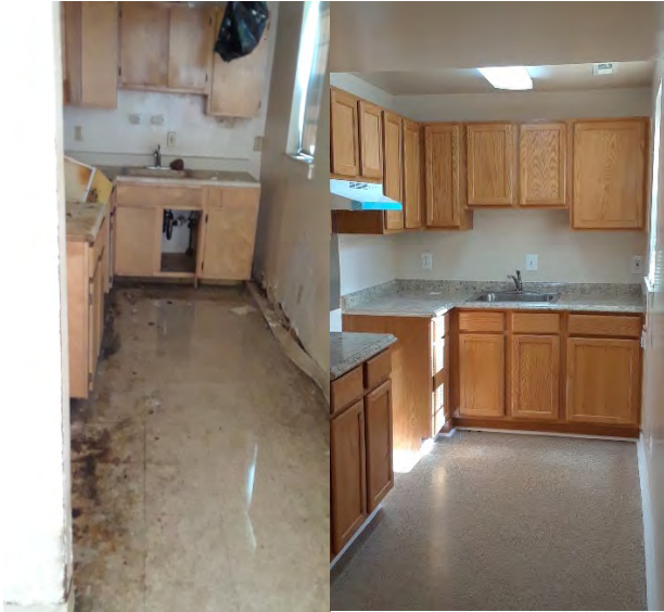
Figure 1. Kitchen at Lincoln Heights, Before and After
