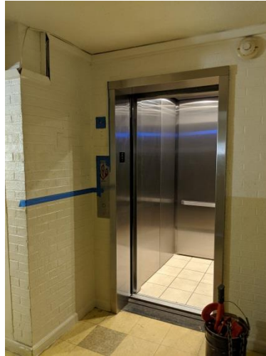
New elevator ready for service
