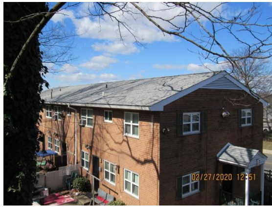
Completed roofs and new windows at Stoddert Terrace
