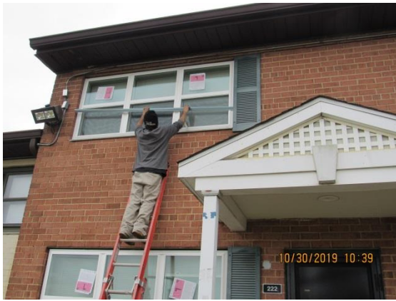
Work underway in October 2019 to replace windows Stoddert Terrace
