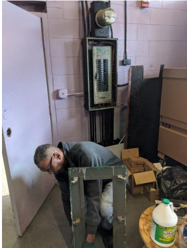
Work underway to replace electrical gear at Potomac Gardens elevator
