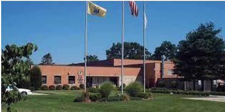
FCI Ft. Dix Administration Building
