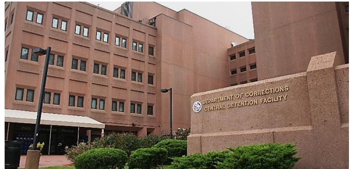
Central Detention Facility (CDF)
