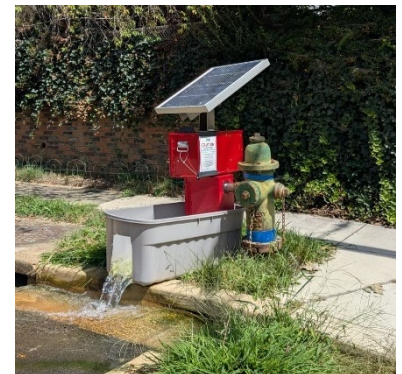
An example of an automated, solar powered flushing device.
